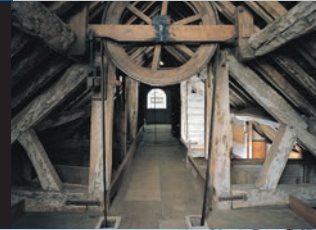
The attic floor or garner
